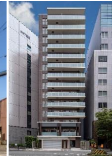
Takamatsu Corp Osaka H Condominium, Toyosaki
