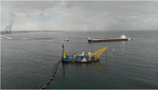
Mirai Construction Hachinohe Harbor Hattaro/Kawaragi District Cruise Path / Anchorage Dredging (Phase 2)
