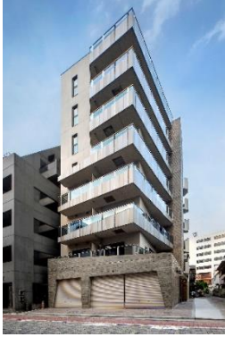
Takamatsu Corp Tokyo S Building, Shiba
