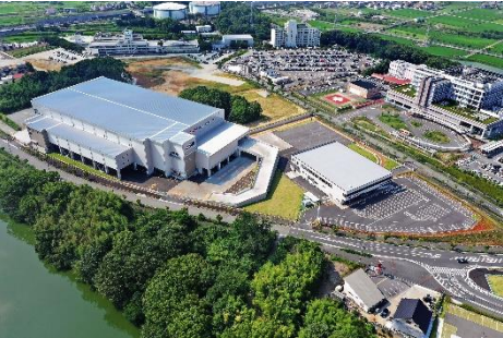
Asunaro Aoki Construction (Temp) Maruai Logistics Center Construction
