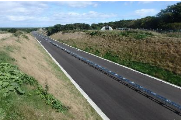
Asunaro Road Route 44 Nemuro City Onne-toh East Pavement
