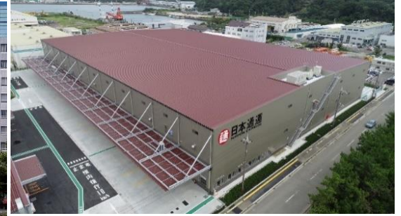
Takamatsu Corp Osaka Nippon Express Co.,Ltd. Wakayama Warehouse
