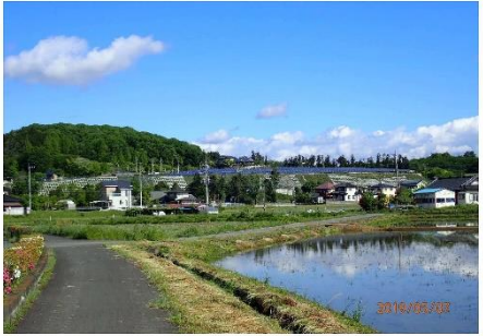
Toko Geotech Tohoku Highway Slope Repair / Construction Between Tochigi-Tsuga JCT and Kanuma Interchange
