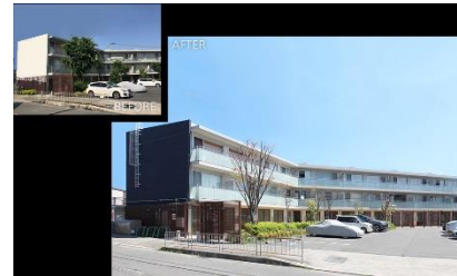
Takamatsu Techno Service (Osaka) Outer Wall Refreshing, RC 3 Floor Building
