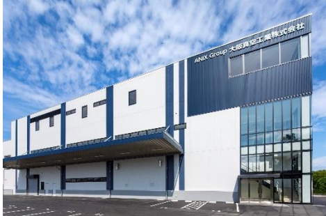
Asunaro Aoki Construction (Temp) Osaka Vacuum Industrial Co.,Ltd. Hoshida Plant Construction
