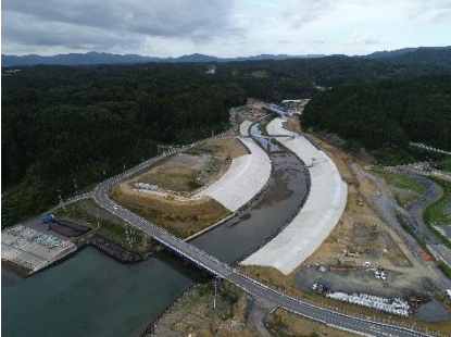
Asunaro Aoki Construction Isato-Maekawa Recovery Construction (Phase 2)
