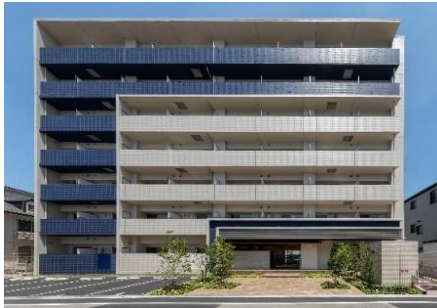
Takamatsu Corp Osaka Company O Dormitory, Hanaten
