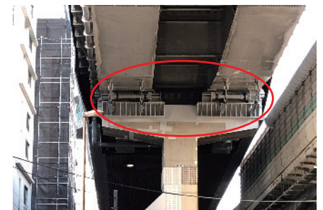
"Die and Rod Type Friction Damper" installed on the Daiba Line of the Tokyo Metropolitan Expressway
