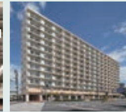
Photo 5. Installation of seismic control brace (entire view)
