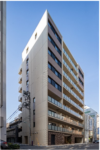
Takamatsu Corporation Higashi-nihonbashi / condominium new construction
