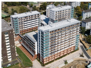
Asunaro Aoki Construction 29-Shinsenri Higashimachi housing complex construction work
