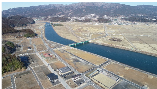
Asunaro Aoki Construction 2015 Takata district & Imaizumi district residential land maintenance Other construction
