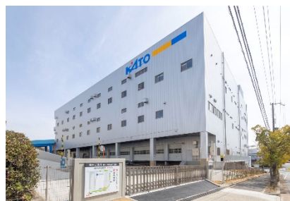
Asunaro Aoki Construction KATO SANGYO CO., LTD. Nishi-kinokuni Division Shinko branch new construction work
