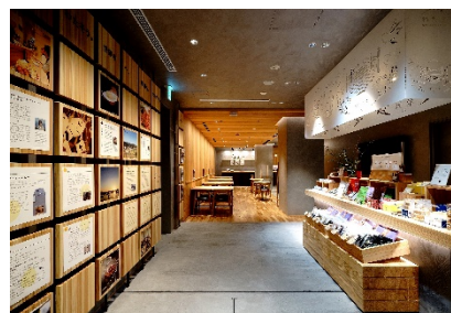
M's "Watasu Nihonbashi" Nihonbashi Mitsui Tower 2nd floor move-in work
