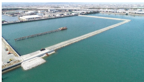
Mirai Construction Yatomi Wharf No. 1 Revetment on the north side Maintenance work (1)
