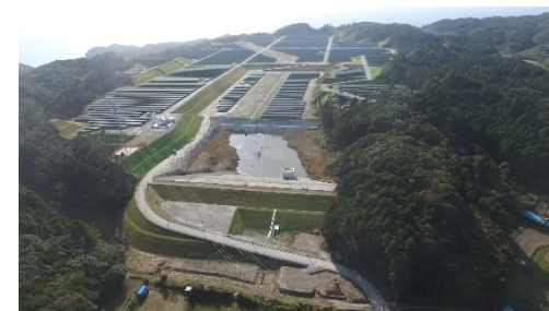
Asunaro Aoki Construction Katsura City Okitsu Solar Power Plant Construction Work (Civil Engineering Work)
