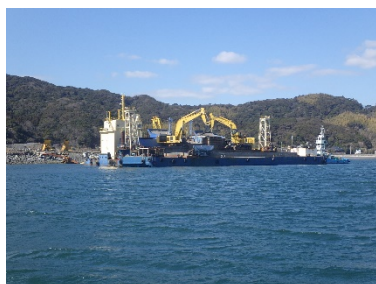
Aoki Marine Fukuyama Port Minooki area revetment (-10m) construction work(Part 2)
