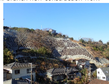
Toko Geotech FY2020 steep slope collapse countermeasure construction (public)Part 1
