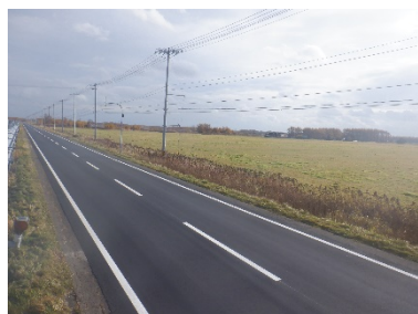
Asunaro Road Nakashibetsu Shibecha Line pavement (structural improvement) Construction Nakashibetsu branch office construction site
