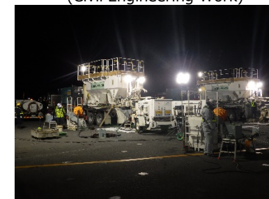
Toko Geotech FY2020 Tokyo International Airport C runway, etc. Ground improvement work
