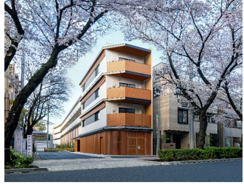
Takamatsu Corporation Ekoda / condominium new construction
