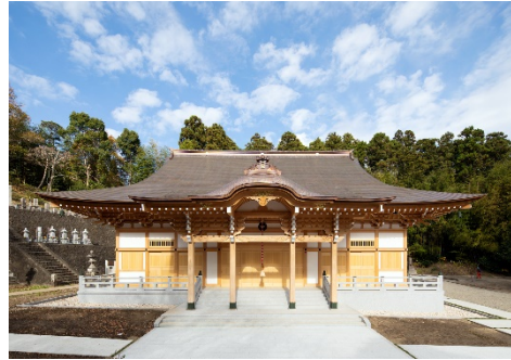
Kongo Gumi Jyusenji main temple new construction
