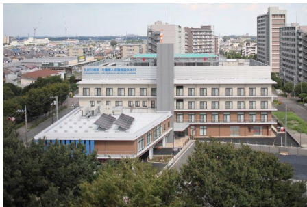
Asunaro Aoki Construction New construction of Kumegawa long-term care health facility (tentative title)
