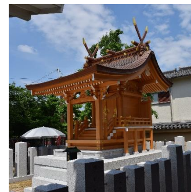
Kongo Gumi (Tennoji-ku, Osaka) New construction of Shitenno-ji Yomeiden
