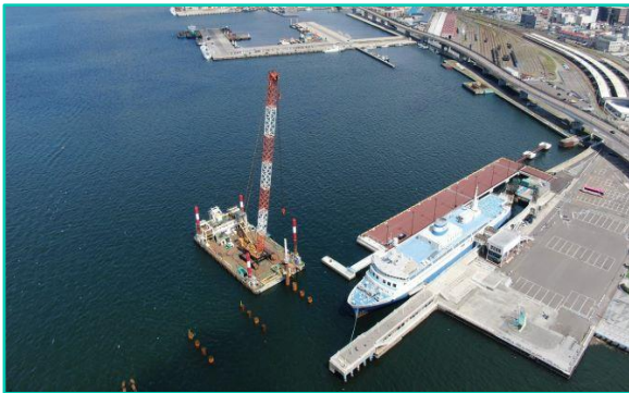
Quay wall improvement work in the Hakodate Port Wakamatsu District
