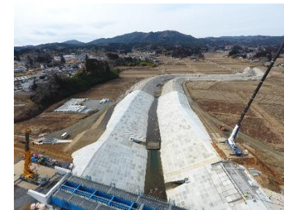
Asunaro Aoki Construction Okinota River flood damage recovery work (3)
