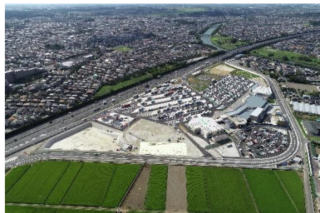
Asunaro Aoki Construction Construction of Tohoku Expressway Hasuda Service Area (inbound)
