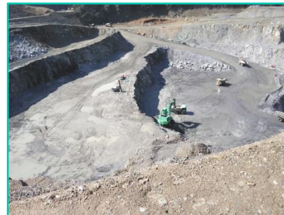
Koishiwara River Dam work (blasting work)
