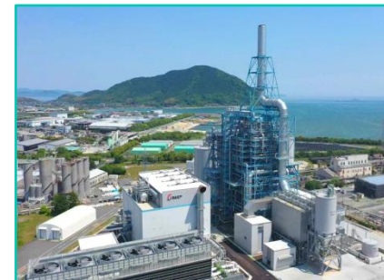
Hofu Biomass Power Plant construction (insulation/heat-resistance work)
