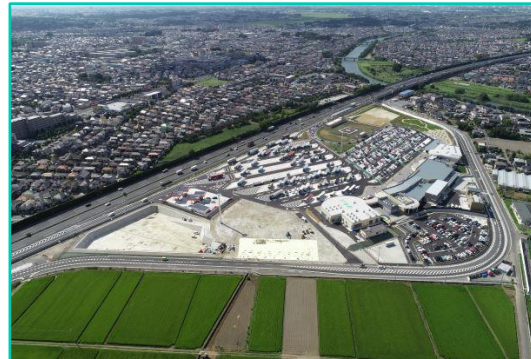
Construction of Tohoku Expressway Hasuda Service Area (inbound)
