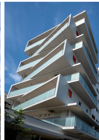
Takamatsu Corporation Osaka Suita, condominium
