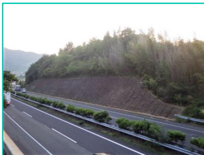
Kagawa expressway slope repair work (slope protection work)
