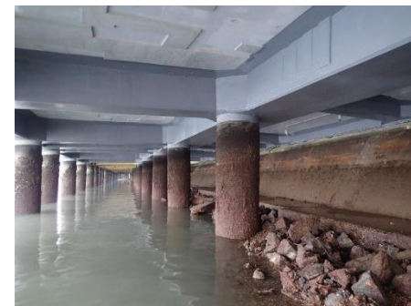
Toko Geotech National Route 185 Sando Bridge repair work #2
