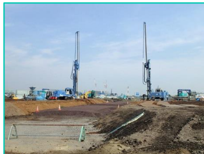
Haneda Airport site foundation maintenance work (ground reinforcement work)
