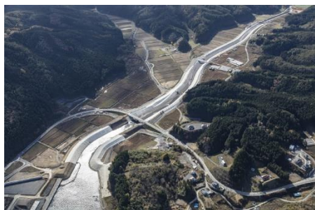
Aoki Marine Mitobe River adjacent area disaster recovery work
