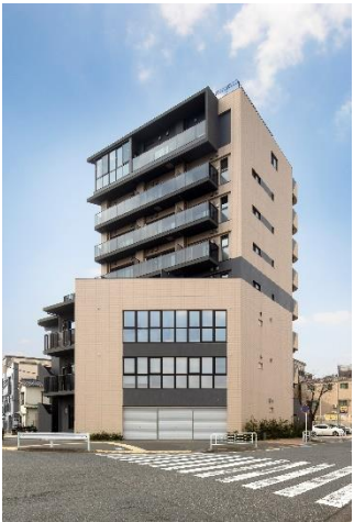
Takamatsu Corporation Tokyo Shiomi, condominium
