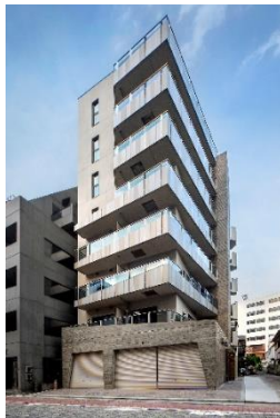
Takamatsu Corp Tokyo S Building, Shiba
