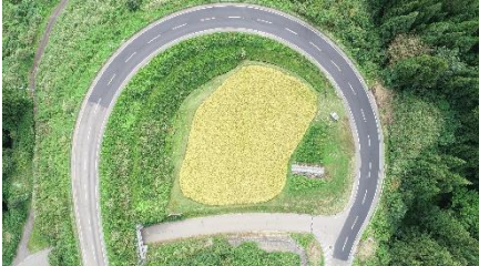
Niigata Mirai Prefecture Road 1201-00-00-05 (Main) Tokamachi Tokan-Shiozawa Road Pavement
