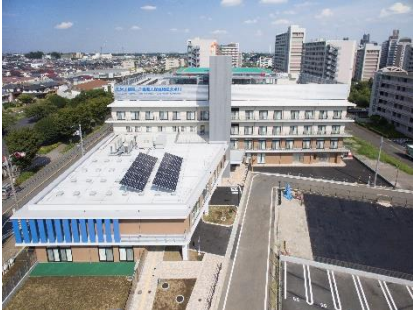
Asunaro Aoki Construction (Temp) Senior Citizen Nursing Facility Construction, Kumegawa
