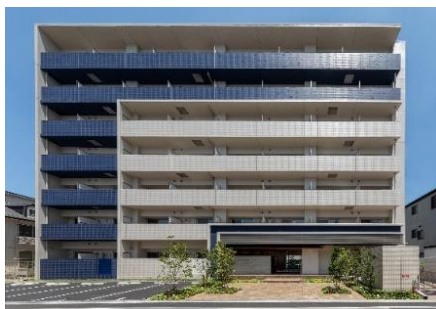
Takamatsu Corp Osaka Hanaten O Dormitory
