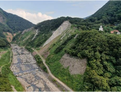
Toko Geotech Lower Portion of Kuzuha Ridge Construction Phase 12
