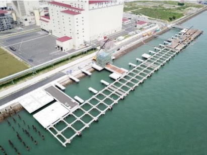
Mirai Construction Mizushima Tamashima District Wharf (-12m) Construction (Phase 4)
