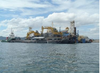
Aoki Marine Mizushima Harbor Tamashima District Wharf (-12m) Dredging Construction
