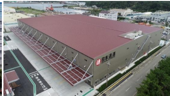
Takamatsu Corp Osaka Nippon Express Co.,Ltd. Wakayama Warehouse
