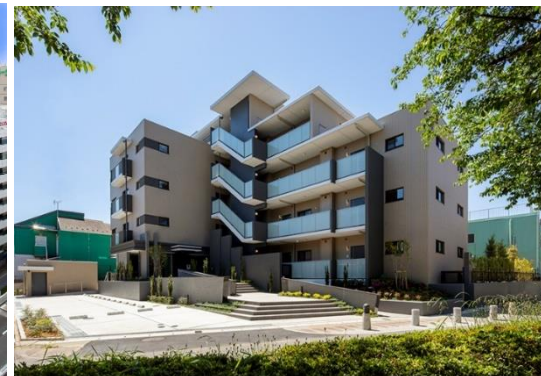
Takamatsu Corp Tokyo W Condominium, Urayasu
