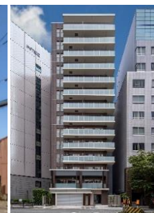
Takamatsu Corp Osaka H Condominium, Toyosaki
