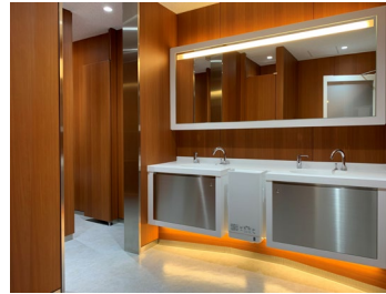
M's NBF Shibuya East Building Toilet repair work
