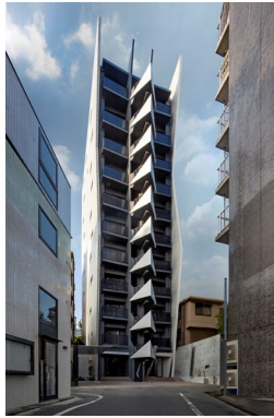
Takamatsu Corporation Near Yoyogi koen station New construction of "FELICE Yoyogi koen"
