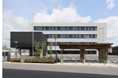
Asunaro Aoki Construction Tochigi Regional Joint Government Building (FY2018) Construction work
