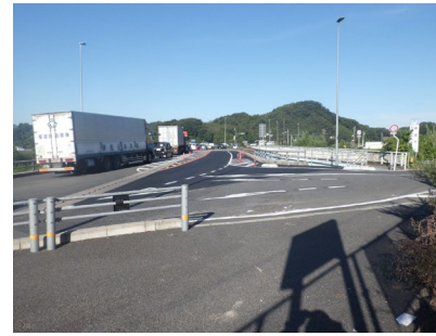
Toko Geotech National highway No. 2 Hasegawa Bridge Outer bridge repair work
