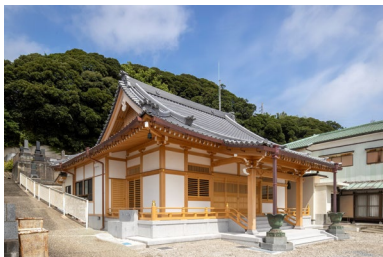
Kongo Gumi New construction of Houzen-ji main hall in Yokosuka
