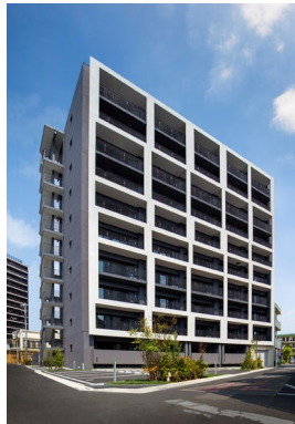
Takamatsu Corporation In Warabi New construction of Fusou limited company's condominium
