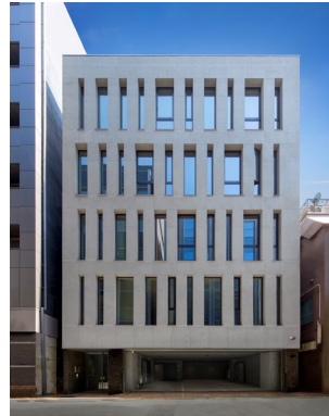
Takamatsu Corporation In Ginza New construction of Yamakatsu building
