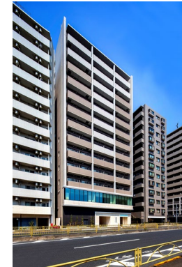
Takamatsu Corporation In Tachiaigawa New construction of Oi Transportation Co., Ltd.'s condominium
