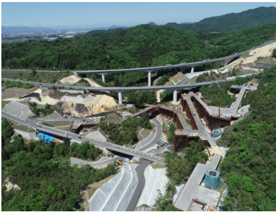
Mirai Construction Shin-Meishin Expressway Kamitanakamimaki construction
