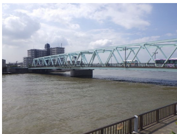
Aoki Marine Honokudo Bridge repair work (pier reinforcement) No.2
