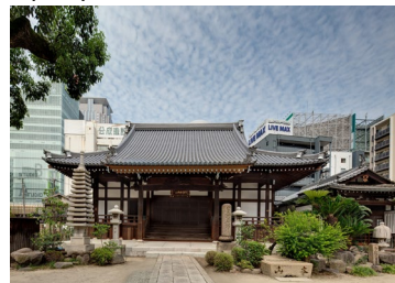
Kongo Gumi Repair work of Genko-ji main hall
