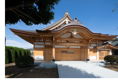
Kongo Gumi New construction of Fukusho-ji main hall
