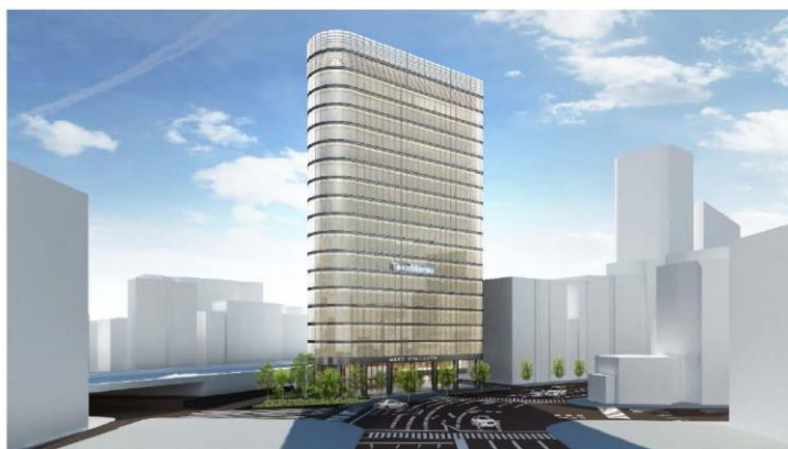
"TCG Building" (tentative name) under construction in Shiba, Minato-ku, Tokyo Number of floors : 18 floors above ground, 1 floor below ground Scheduled start of construction : September, 2020 Scheduled for completion : February, 2023 (Schedule) Main environmental certifications, etc. : Acquired CASBEE A rank Construction : Joint venture between Asunaro Aoki Construction Co., Ltd. and Takamatsu Corporation
