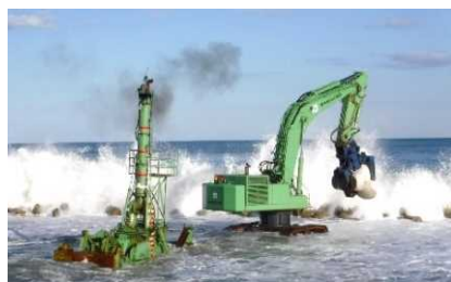
River and coastal construction using amphibious bulldozers, etc.
